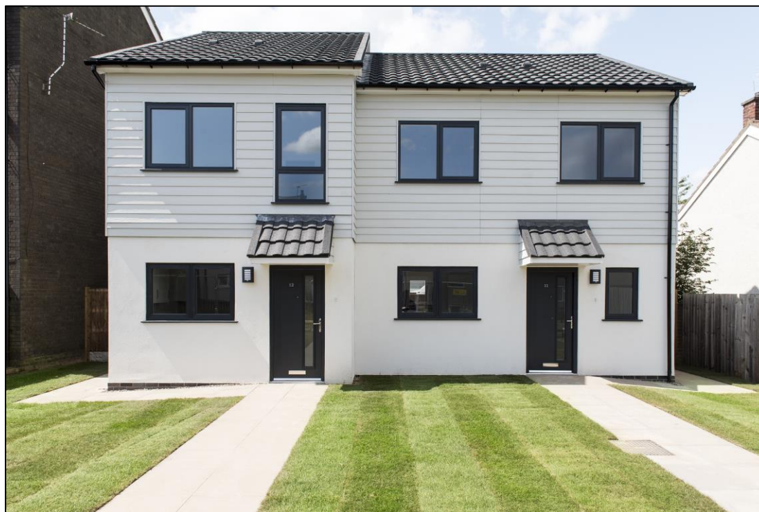
Modular housing delivered at Littlethorpe, Coventry by Citizen Housing (image courtesy of Citizen)
